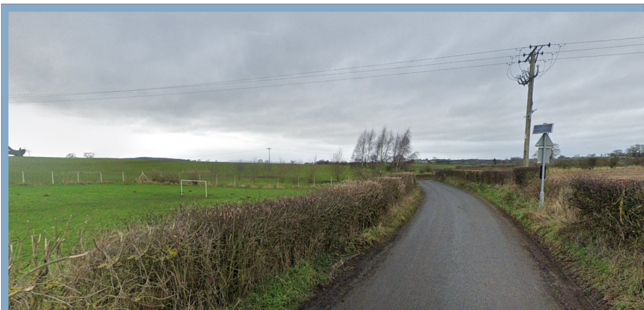
Figure 7-3 Existing powerlines above the playing field and utility pole on side road
